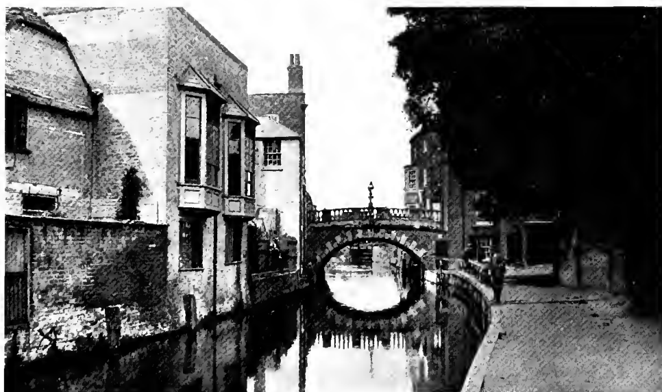
BRIDGE AT NEWBURY, BERKS
